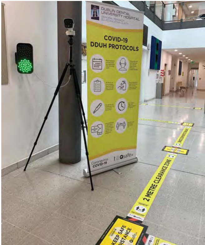
Automatic temperature monitoring has been installed at the entrances to the DDUH.
